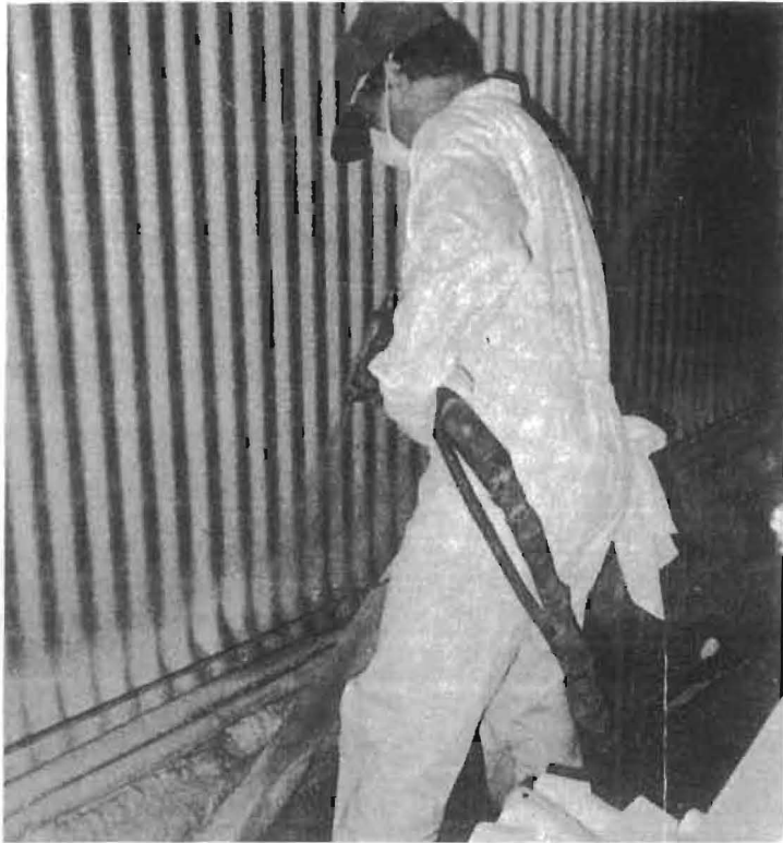
Photo 9. Application of foam inside a horizontal storage.
