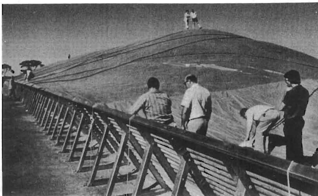
Photo 20. Bunker storage at Wyalkatchem showing the bulkhead type side walls constructed of portable steel frames.
